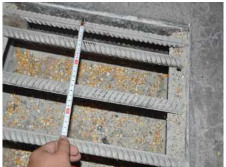
Size check of flap's grid at the grain terminal
